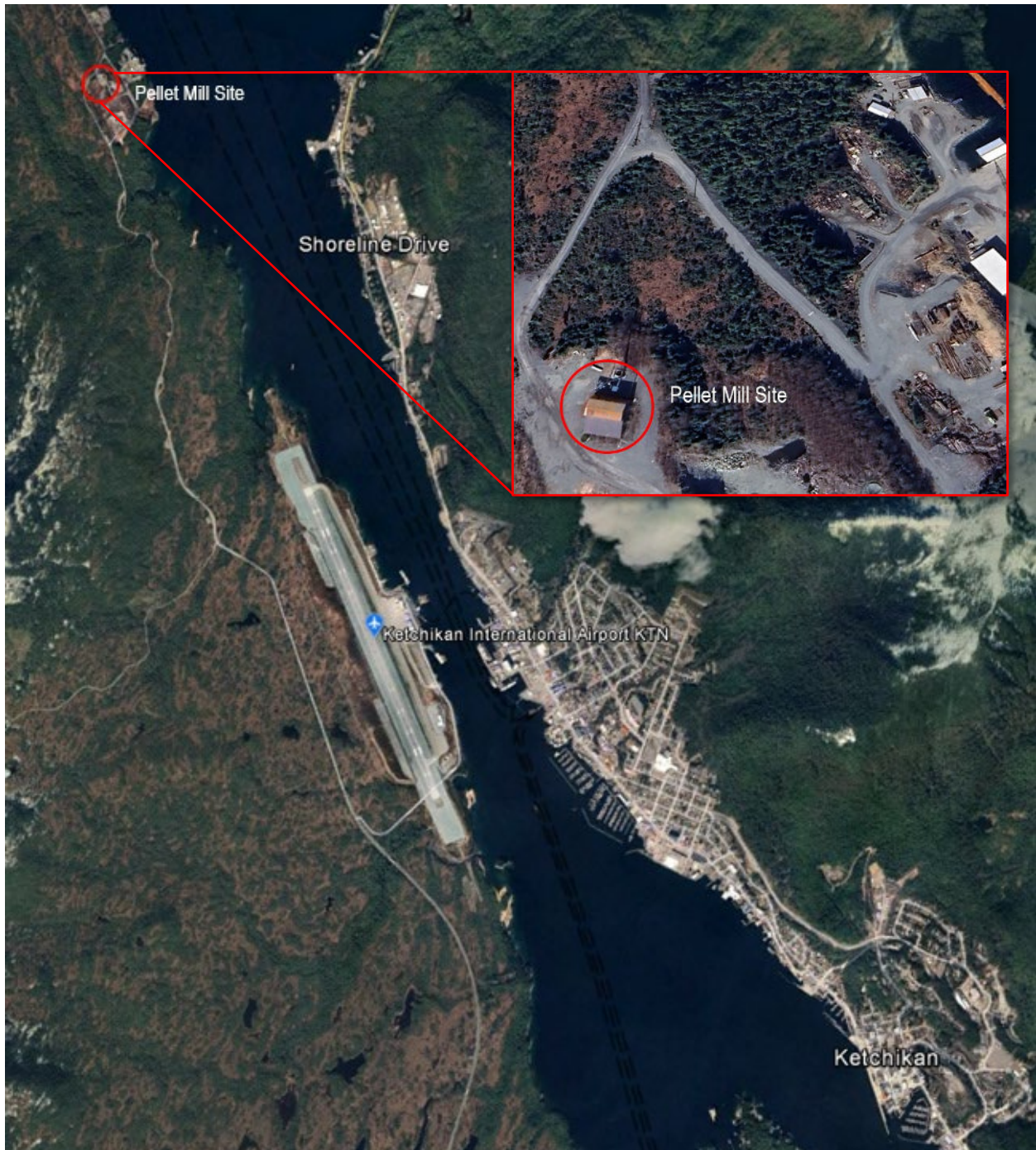
Figure 2. Aerial Image of Ketchikan and the Pellet Mill Site
